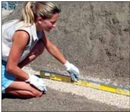
After filling the trench, compact and check for level.
