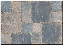
TJP paver use a different type of spacer than what is typically used to create the joint space between pavers. TJP could be installed as a non -permeable pavers in that the joint width is 4.5mm and will accept most stabilized joint sands.
