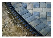
Install 1" of bedding conforms to ASTM C33. This
